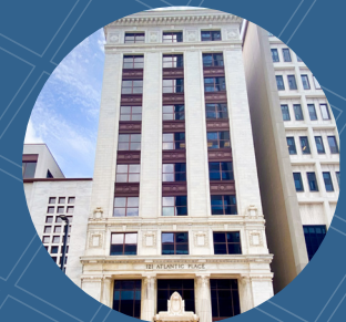
121 Atlantic Building 114,779 SF
